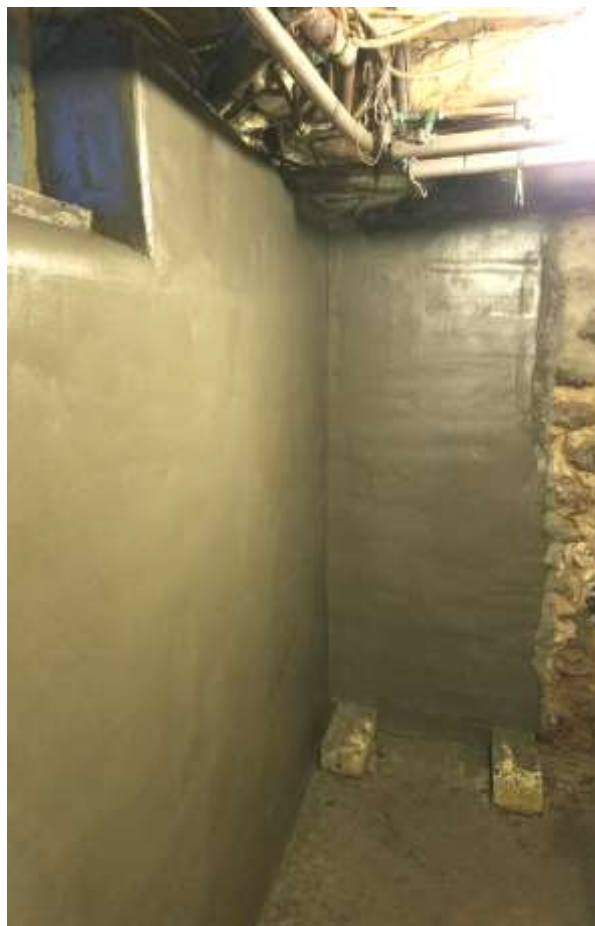
Example Xypex Megamix II over concentrate installed on stone wall.
